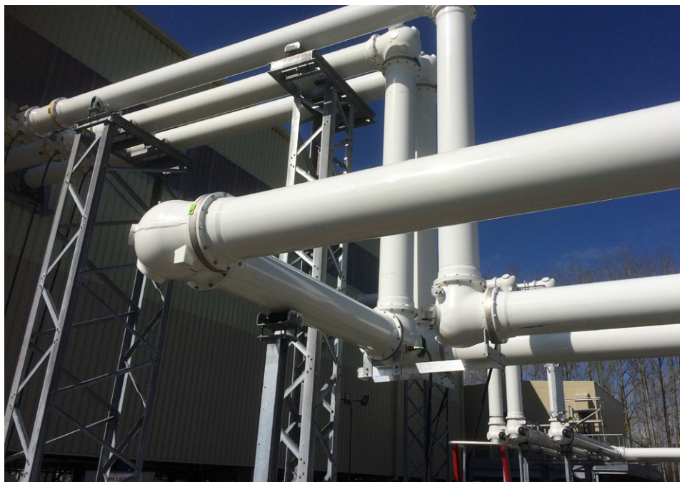
Gas-insulated busbar containing g 3 at Sellindge
