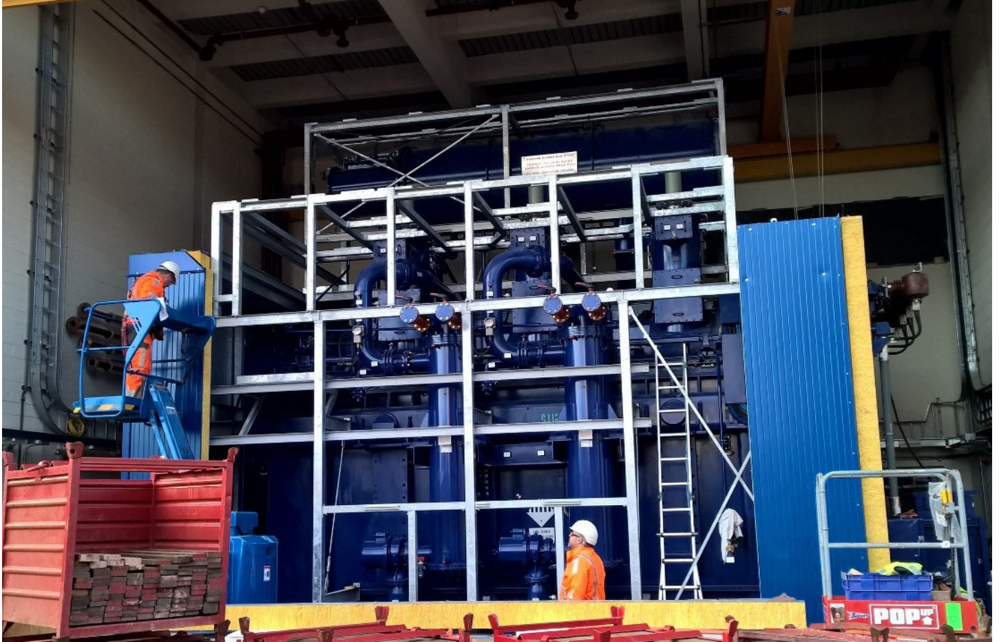
Supergrid transformer containing a synthetic ester
